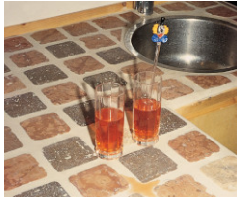
An example of a bonded and grouted kitchen worktop
